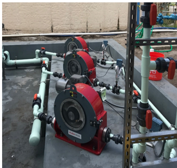
Figure 1. Flowrox single roller design peristaltic pumps hoses lasted approximately 9 months and survived in excess of 11 million revolutions while pumping abrasive lime slurry.
