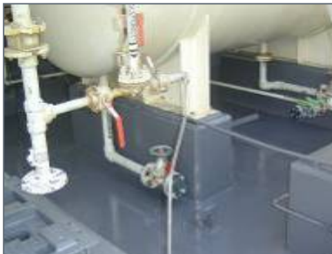
Rebuilt and protected floor
