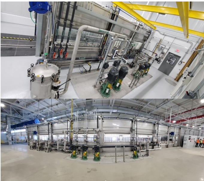
Figure 5. PSI VTPs with Thrust Head design installed at Detroit automotive plant.
